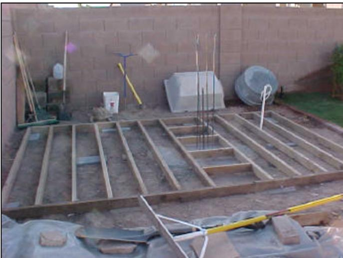
The floor frame. Joists are 1' on center, except around the pier. It rests on the cinderblock "caps" bought at Lowe's. Under suggestion, I went and drove rebar into the ground and hooked them to the frame. This was one of the "just in case" things, but better to do it and not need it.
