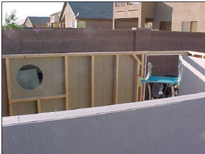
Mount installed on base plate, all 4 walls are up, sided and painted. The hole is for an attic ventilation fan to help maintain ambient temperature during the summer while the roof is closed. It operates on a thermostat so it won't run constantly until it gets hot.
