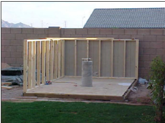
Form tube has been removed, base plate installed, floor laid down, and 2 walls framed. The back wall had the siding installed and painted prior to installation because there's only about 8" between the block wall and the building. The floor is much steadier than I anticipated, and is completely isolated from the pier.
