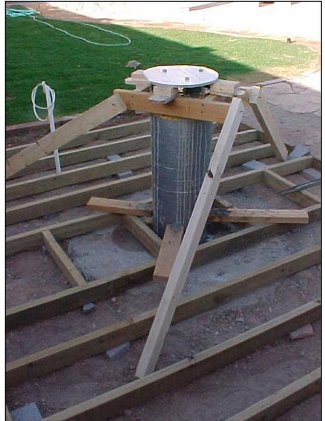
The pier setting up with the J-bolts installed. Took 4 bags and a little to fill the tube to the top. The 2x4 frame up top is for two reasons...to "squish" the tube to 11" in a N-S line to allow room for Zenith viewing, and to provide a platform to hold the J-bolt jig set up. Other than some minor cosmetic issues, it worked like a charm, and I nailed the N/S alignment; with more than enough room for adjustment either direction.
