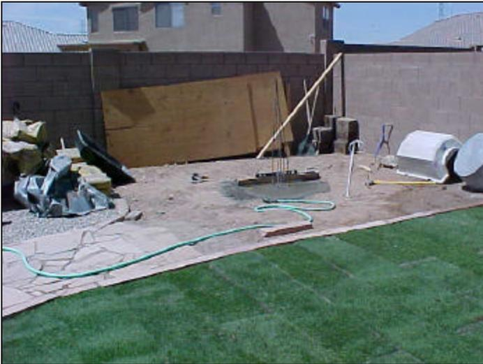
The base for the pier. The hole is 3'x3' by 2' deep, and took 1680 pounds of concrete to fill. Took about 2 hours to mix and pour by myself.
