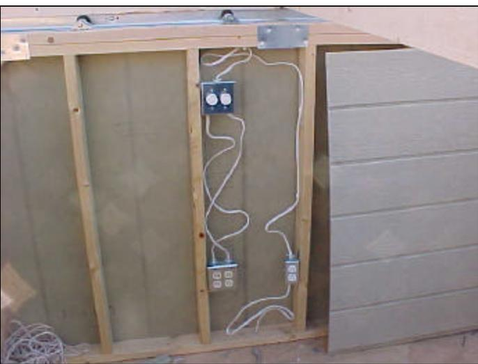
The outlet on the right is for a future computer to be placed in the observatory. The 2 outlets on the left are hooked to the dimmer switches for optimum adjustment of the red lighting which will be plugged in to them. I ended up enlisting the help of a family member to troubleshoot the wiring, which kept tripping the GFI at first. It turned out to be a faulty connection, and not a design issue. There is also a non-dimmed outlet at the base of the pier to plug the 'scope into.
