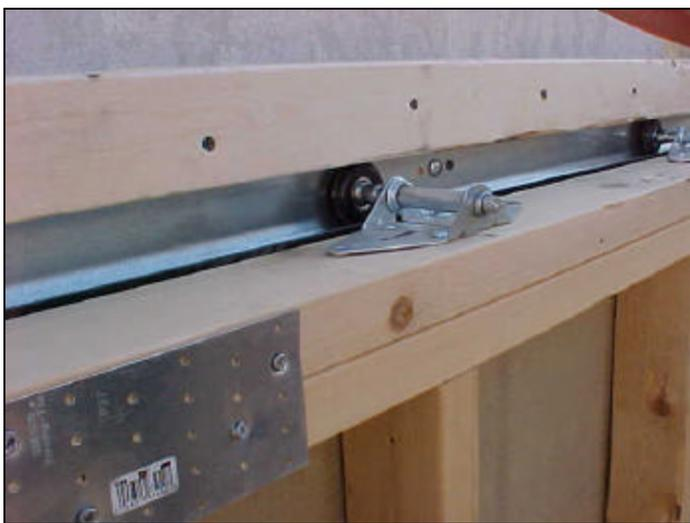
Close up of the rollers and track for the roof. I used garage door rollers and track. The rollers are nylon with ball bearings. I don't have the full roof weight yet, but with 10 rollers total at several hundred pounds capacity each, I don't anticipate any problems.
