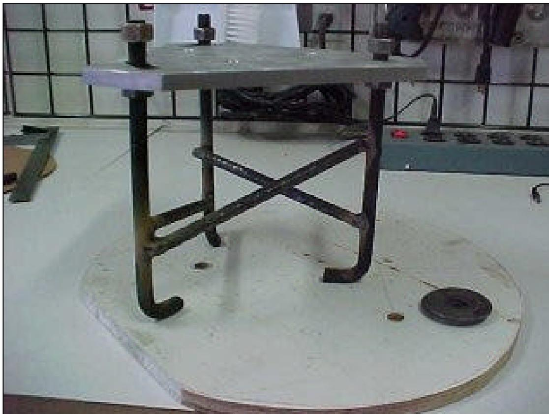
The baseplate is the link between the pier and the telescope's equatorial head. The J bolts will be sunk into the wet concrete, and the plywood circle will hold the j bolts in position while the concrete sets
